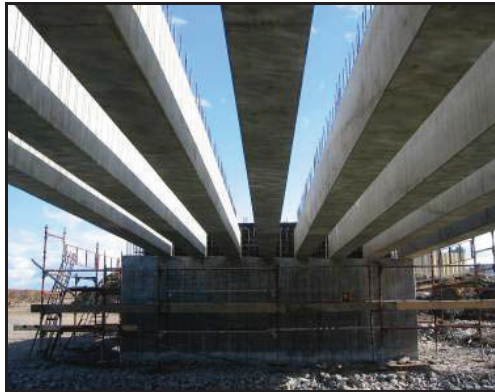
Figure 3.5 Prefabricated beams on top of substructure
