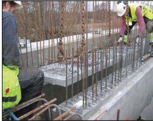
Figure 3.6 Placing prefabricated bridge slabs between beams
