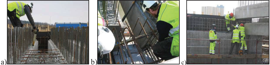
Figure 5: a) Mounting beam. b) Stabilizing edge beam. c) Reinforcement sticking up.
