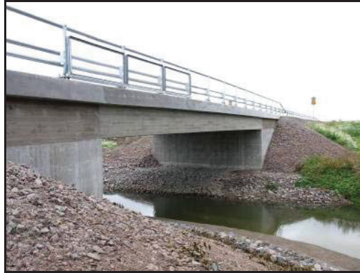
Figure 3.2 Completed semi-prefabricated bridge
