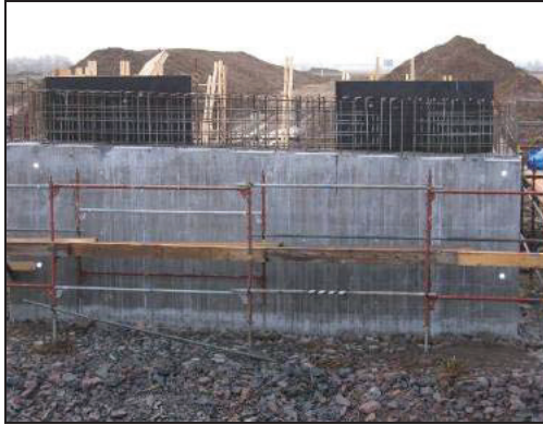
Figure 3.4 On-site constructed substructure
